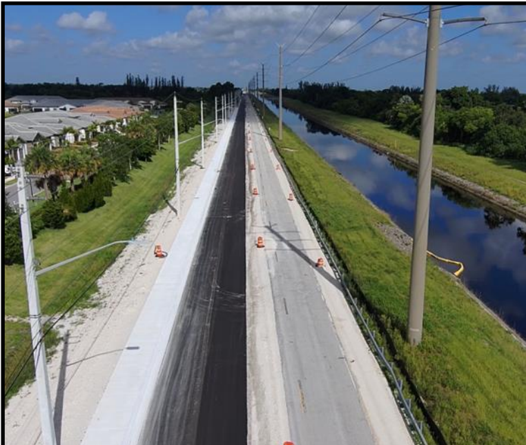
Structural Asphalt Placement
