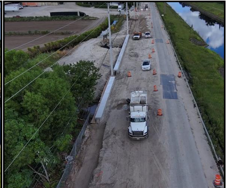
Coping Installation at sheet pile locations
